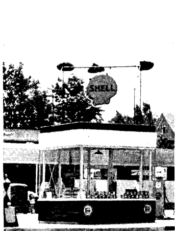
Glass-walled service station
