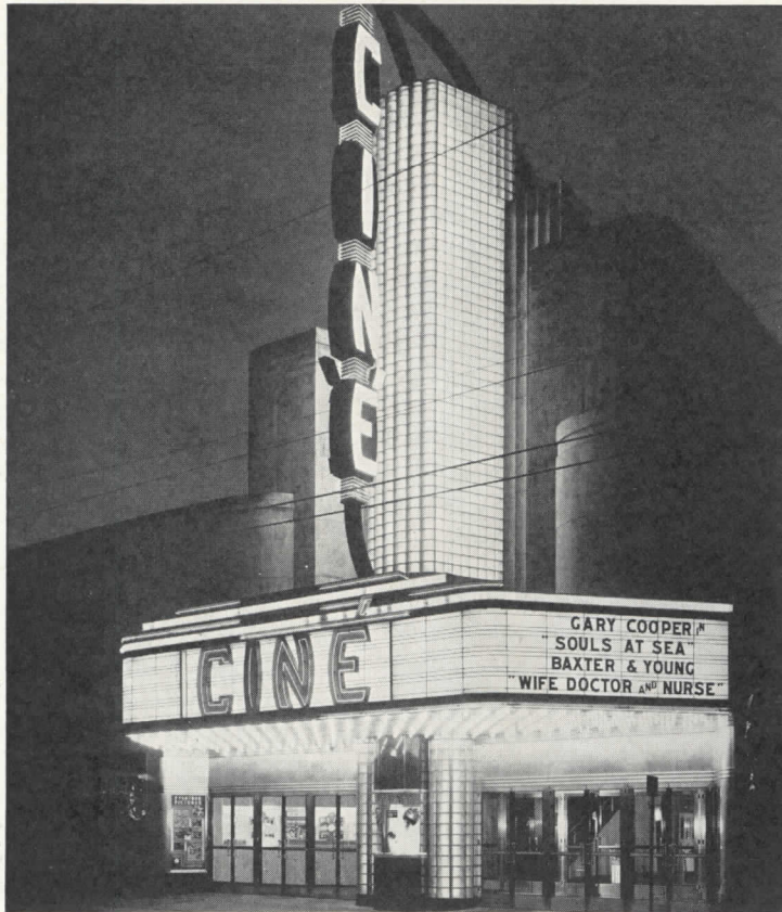
Photo by Hedrick-Blessing. G. W. & George L. Rabb, Inc., architects
