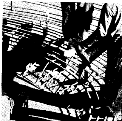
7 Pouring begins; speed is guaranteed by . . . 8 the rotating, rubber hose and . . . 9 rotating screed gets an accurate profile.
