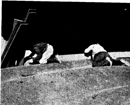
10 Then formwork is removed . . . 11 top surface waterproofed . . . 12 and the underside spray-painted.
