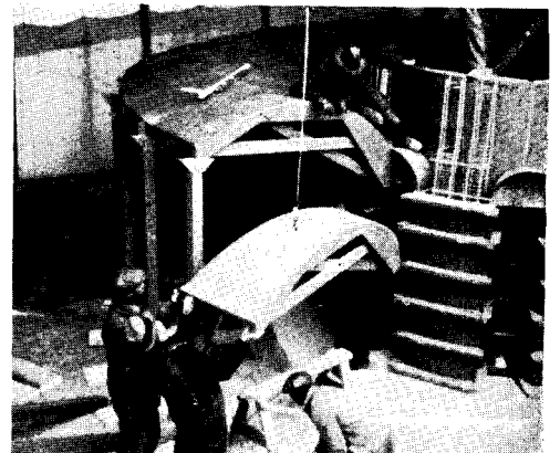
1 Footings are poured, allowed to set and . . . 2 forms are hoisted into place . . . 3 by the derrick which tops the tower.
