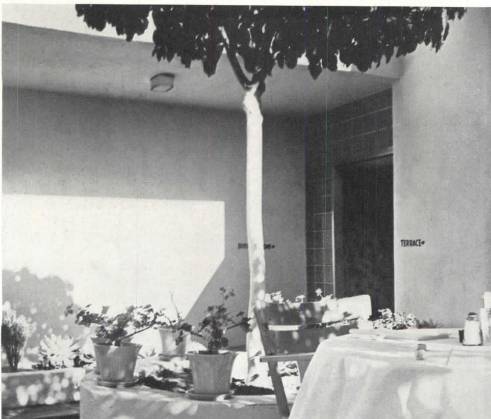
Exterior walls of the restaurant are of groutlock brick; lintels and beams are of reinforced concrete. The over-all finish is white plaster. Footings and floors are concrete; terrace floor is flagstone. Color comes largely from the wide use of potted plants.
