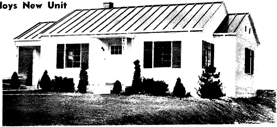
Exterior walls are free of bolts, screws or welding seams.
