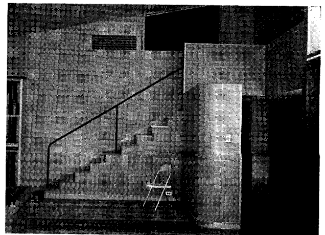
Looking toward service portion
