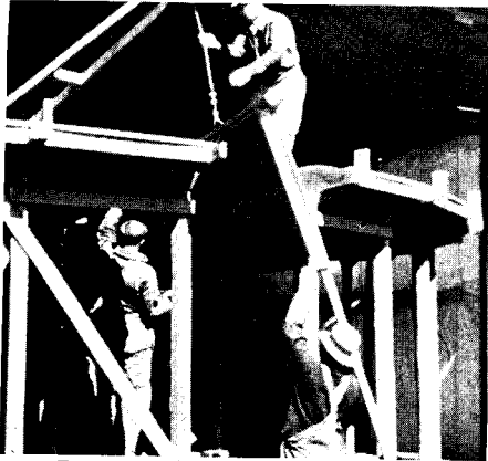
4 Forms in place, reinforcing begins . . . 5 with pre-crimped radial steel; then . . . 6 concentric reinforcing is threaded off.
