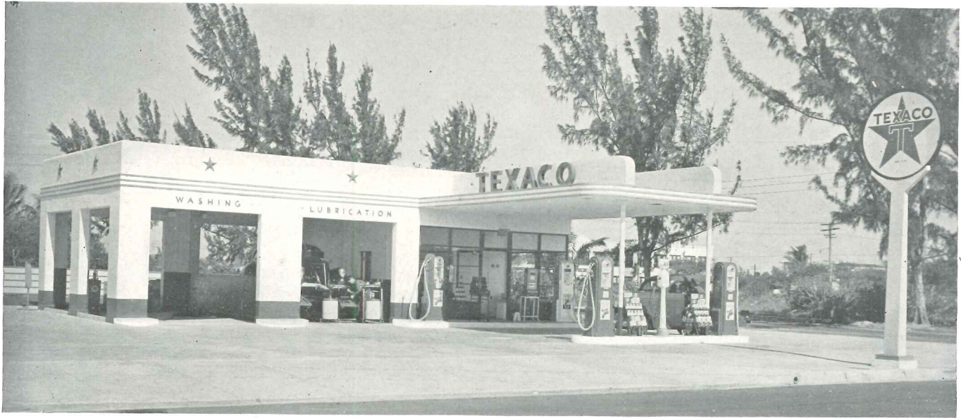
TYPE "C" STATION, canopy addition. Miami, Florida.
