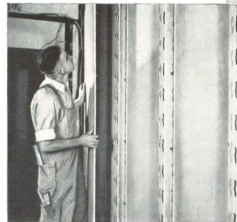
● Concealed steel holding devices and studs form the framework for Transite Walls . . . most modern of movable wall partitions. And this exclusive construction method gives these walls a solidity in keeping with their own inherent durability.
