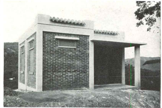
SOME OF PUERTO RICO'S MANY STRAW HUTS HAVE BEEN REPLACED by these modern hurricane-proof houses. Monolithic in construction, designed to resist horizontal wind velocities up to 150 m.p.h., they have flat or nearly flat concrete roofs not subject to wind pressure.
