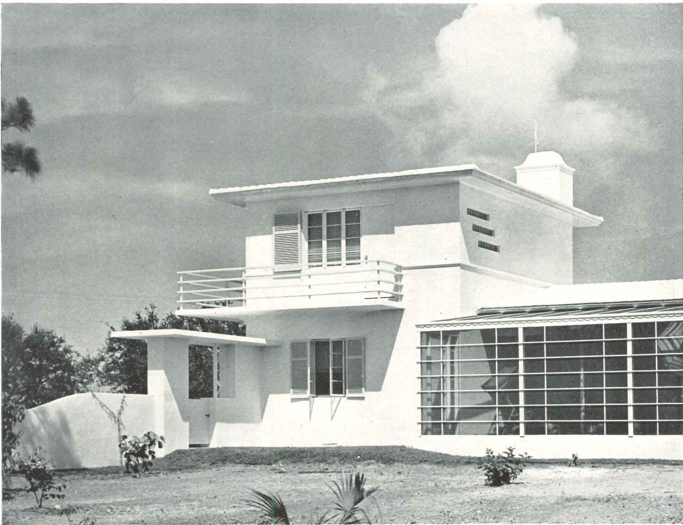
VIEW SHOWING PATIO SCREEN
