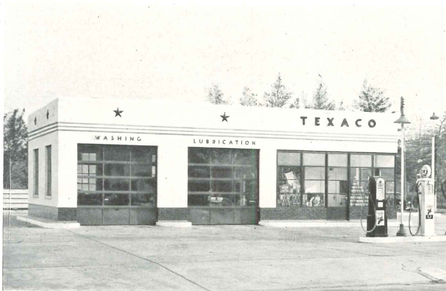
TYPE "D" STATION. Similar to "C" with one lubrication bay, similar office and storage space. Canopy omitted. Norfolk, Virginia.
