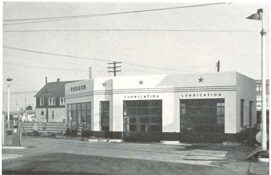
TYPE "B" STATION (for corner lot only). Two bays and office with stucco facing. New Haven, Connecticut.
