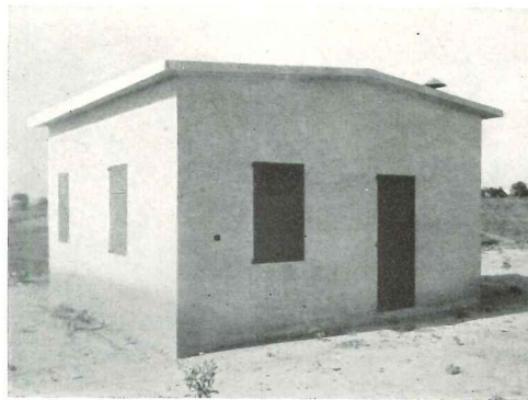
SOME OF PUERTO RICO'S MANY STRAW HUTS HAVE BEEN REPLACED by these modern hurricane-proof houses. Monolithic in construction, designed to resist horizontal wind velocities up to 150 m.p.h., they have flat or nearly flat concrete roofs not subject to wind pressure.
