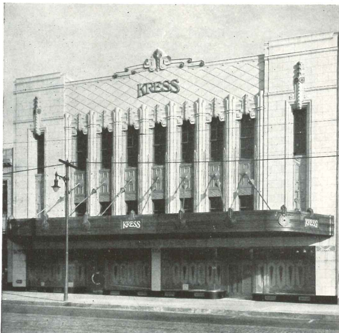
S. H. Kress Co., East Orange, N. J. . . . E. F. Sibbert, Architect Virginia Black Serpentine used for bulkheads.
