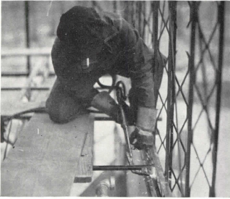
1. Torch instead of saw for cutting.
