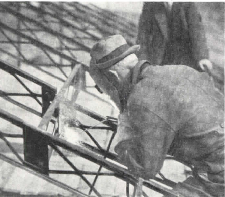
3. Torch replaces hammer and nails.
