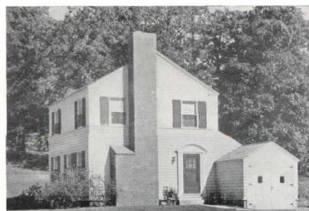
HOUSE NO. 5: An all-wood project sponsored by the National Lumber Manufacturers Association.
