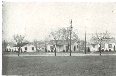
STEEL HOUSES ARE NOTHING NEW TO home owners of the Ohio steel center of Middletown. Here are four built several years ago and right across the street six more are in the process of erection.
