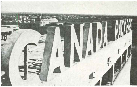
1 The free-standing reinforced concrete sign.
