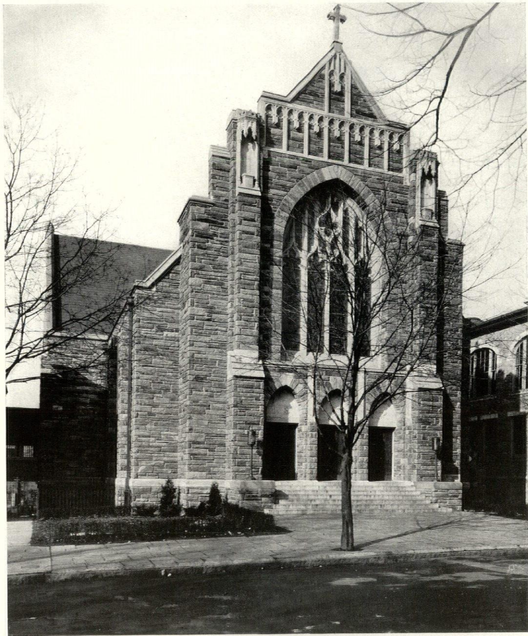
ST. AGNES ROMAN CATHOLIC CHURCH, WEST CHESTER, PENNSYLVANIA Henry Dagit & Sons, Architects
