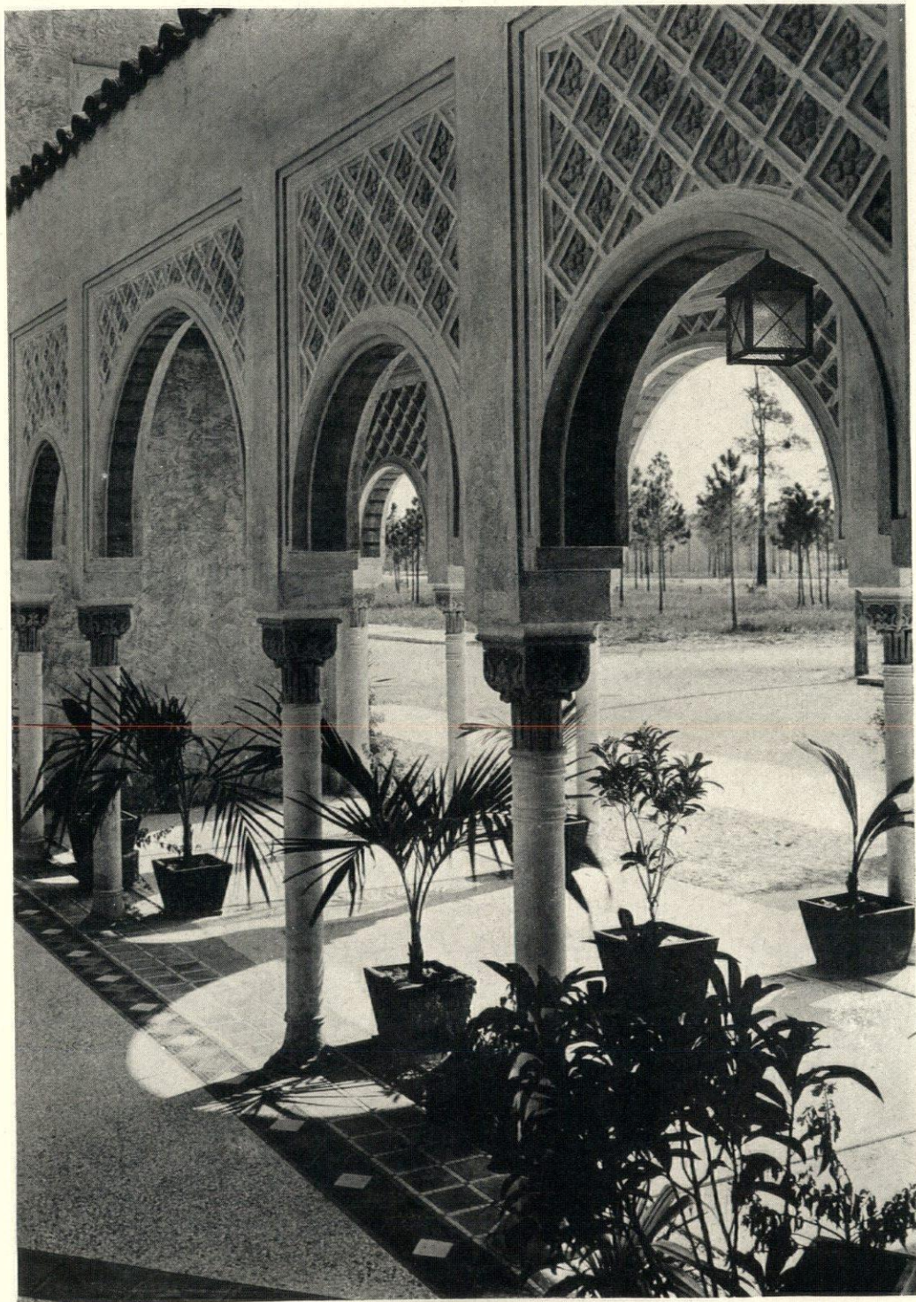
Entrance to Patio CORAL GABLES INN, CORAL GABLES, MIAMI, FLORIDA M. L. Hampton, Architect
