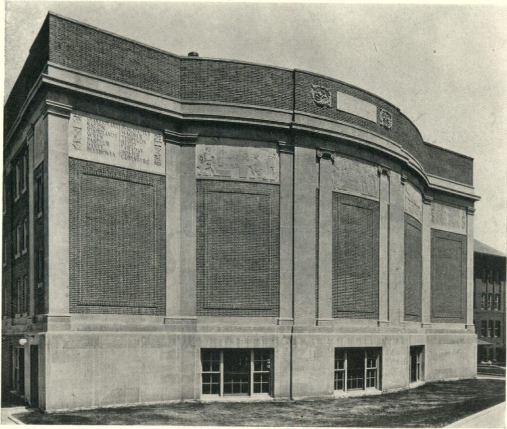
End of Auditorium, Showing Allegorical Panels THE HIGH SCHOOL AT BROOKLINE, MASS. Kilham, Hopkins & Greeley, Architects
