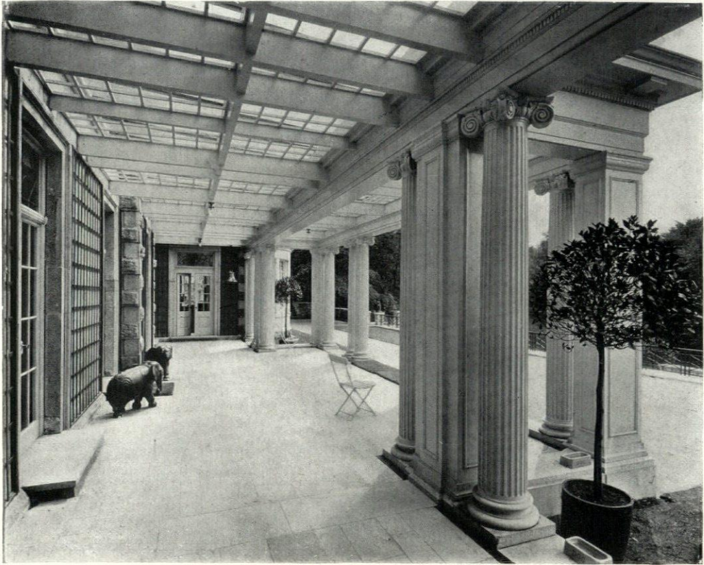
Inside of Verandah "HAZELWOOD," THE RESIDENCE OF W. J. SHARP, ESQ., AT SILVERDALE LANCASHIRE, ENGLAND
