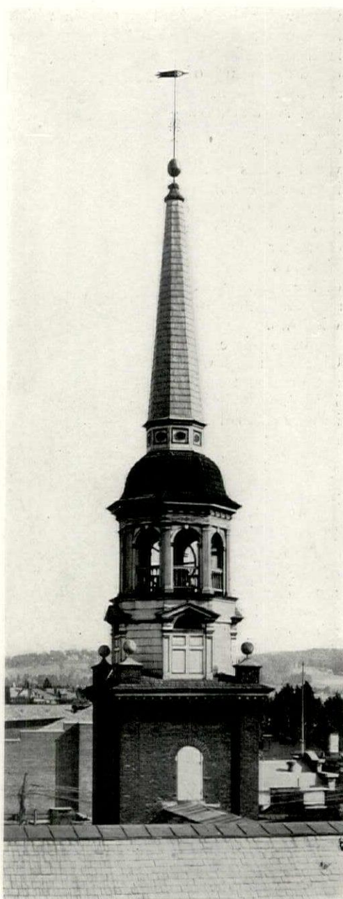
ZION'S REFORMED CHURCH, YORK, 1793-1800. BUILT BY PETER AND JACOB SCHMAHL, DEMOLISHED IN 1913.
