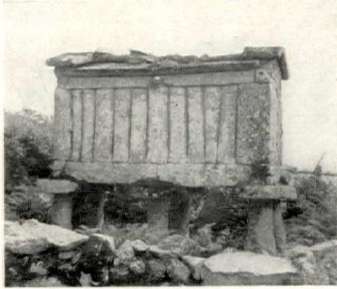
VERY ANCIENT CORNCRIB, NOW ABANDONED; GRANITE ROOF SLABS ARE NINE FEET LONG.
