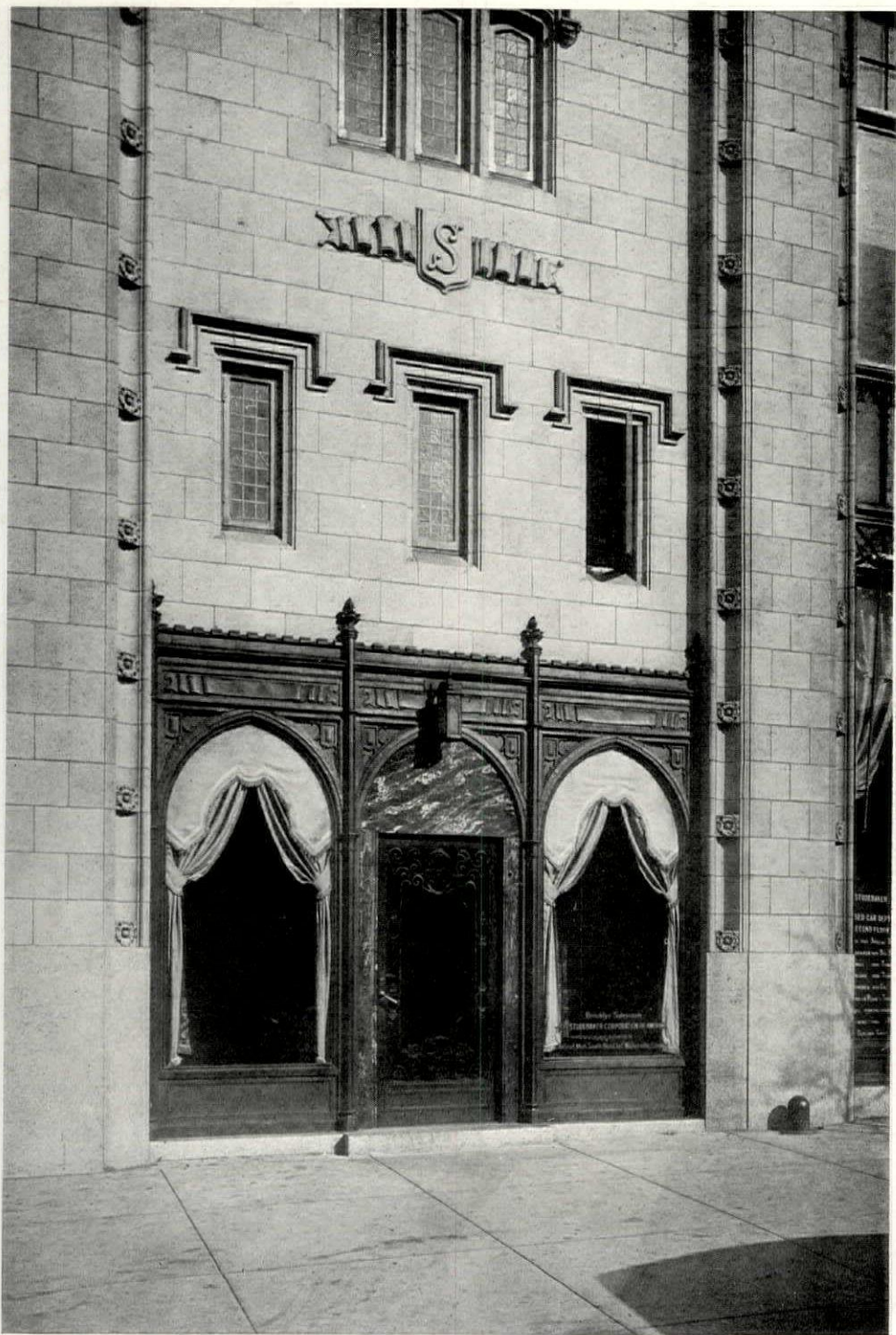
ENTRANCE—STUDEBAKER BUILDING, BROOKLYN, N. Y. TOOKER & MARSH, ARCHITECTS.
