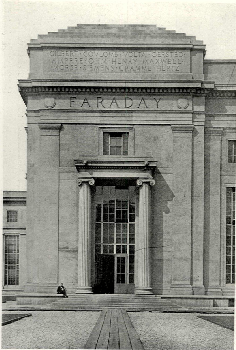
DETAIL—BUILDING FOR THE MASSACHUSETTS INSTITUTE OF TECHNOLOGY, CAMBRIDGE, MASS. WELLES BOSWORTH, ARCHITECT.
