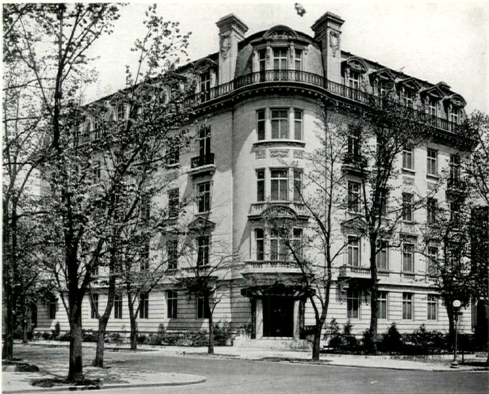
FIG. 130.—APARTMENT HOUSE AT 1785 MASSACHUSETTS AVENUE, WASHINGTON, D. C. J. H. De Sibour, Architect.
