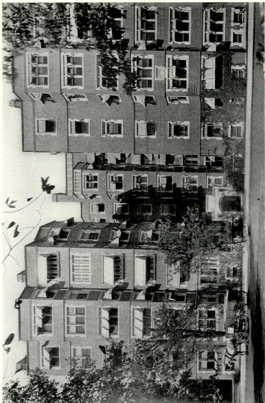
FIG. 136.—MATHER COURT, CAMBRIDGE, MASS. NEWHALL & BLEVINS, ARCHITECTS.
