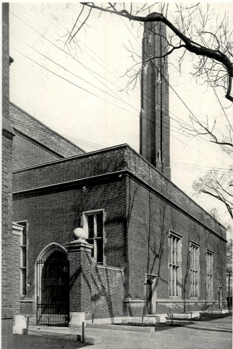
YALE POWER HOUSE, NEW HAVEN, CONN. DAY & KLAUDER, ARCHITECTS.
