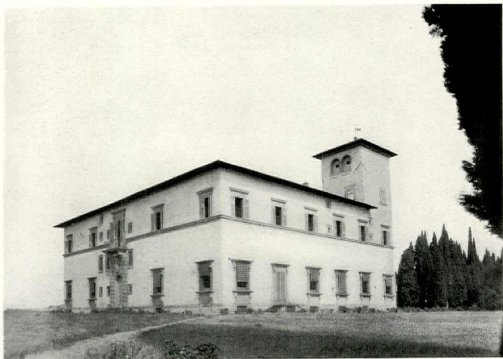
SOUTH AND WEST FRONTS—LE CORTI, NEAR SAN CASCIANO, VAL DI PESA, ITALY.
