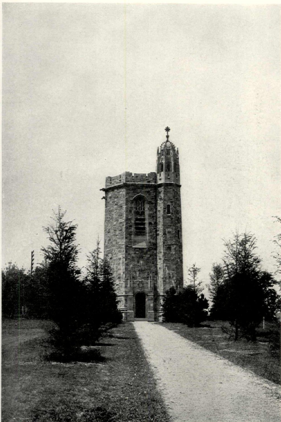
WATER TOWER—CEMETERY OF THE GATE OF HEAVEN. C. W. LEAVITT, ARCHITECT.
