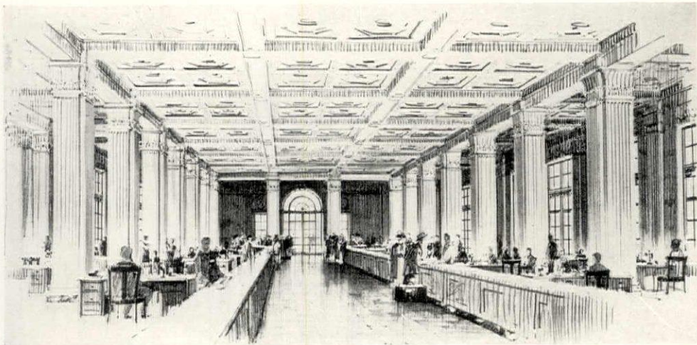
OFFICE SPACE—PHILADELPHIA LEDGER BUILDING, PHILADELPHIA, PA. Arnold W. Brunner, Architect.
