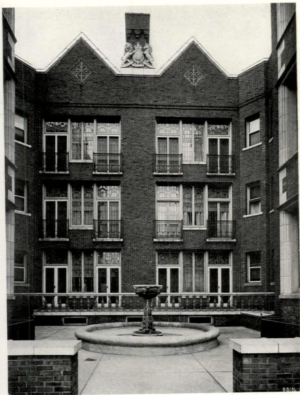
FIG. 91. INTERIOR OF COURTYARD.
