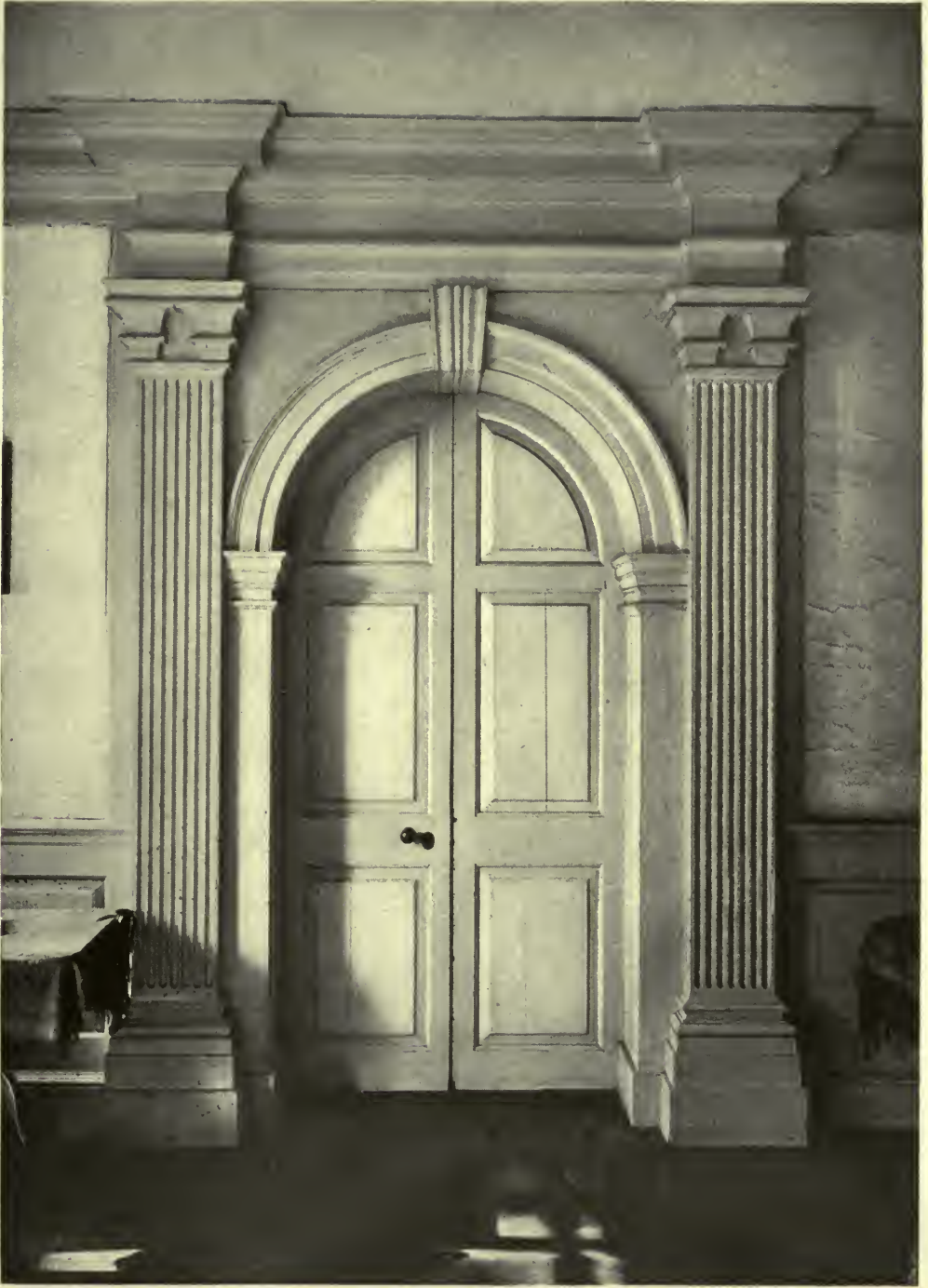
DOORWAY IN HALL—HOPE LODGE, WHITE MARSH, PA. 1723.
