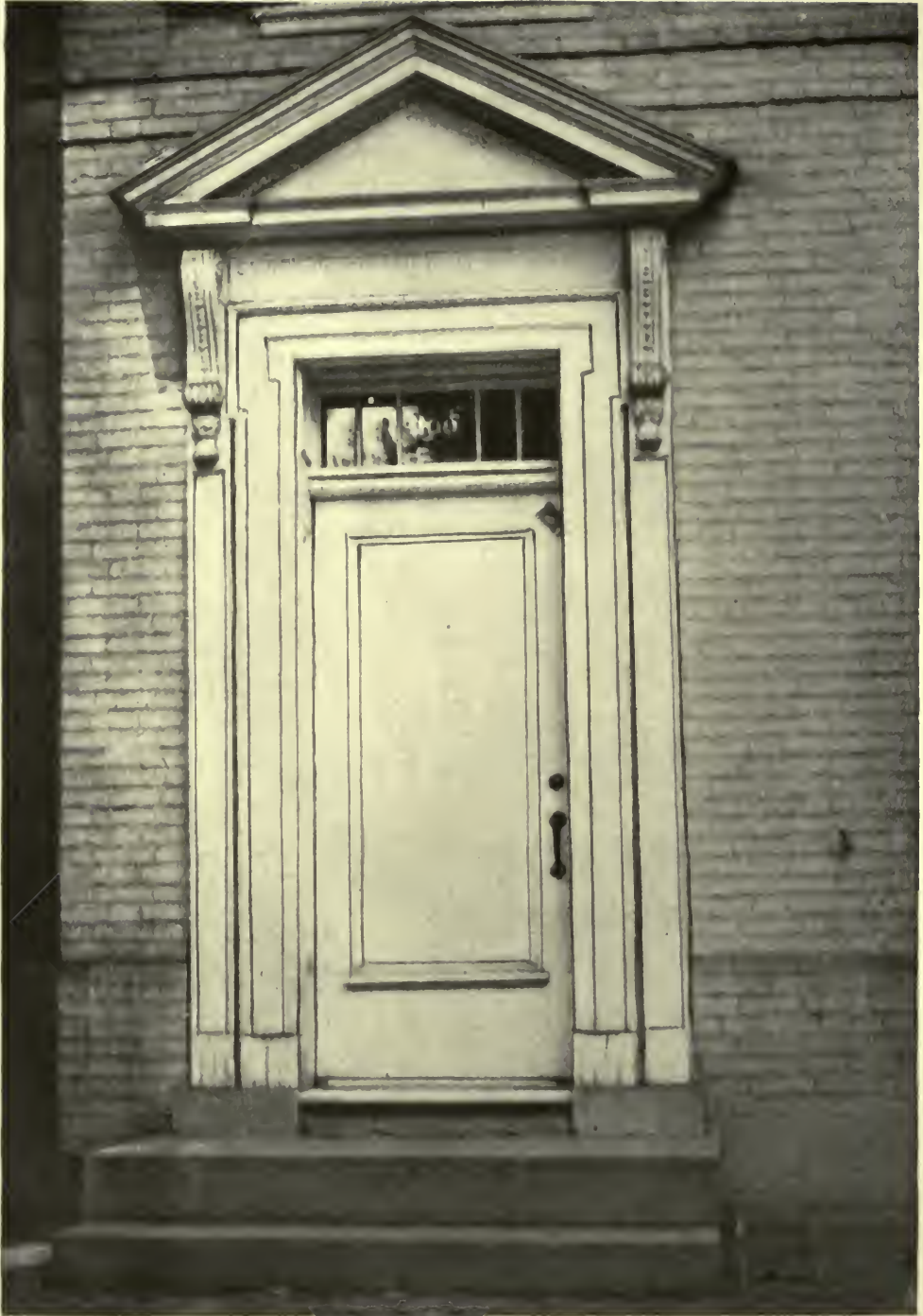
DOORWAY ON FRONT STREET, HARRISBURG, PA.
