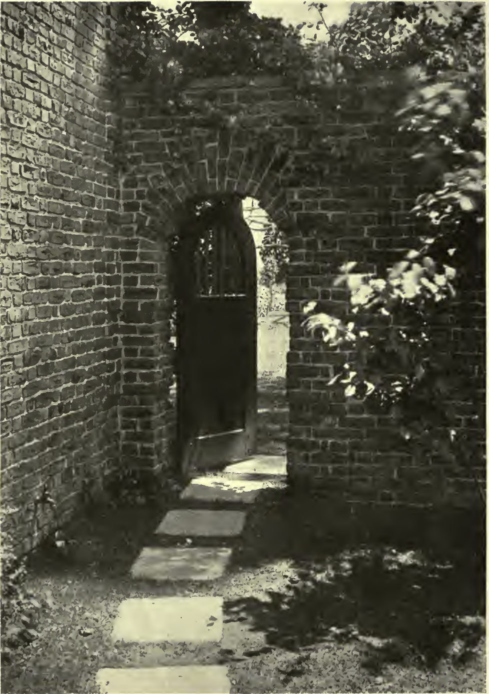
GATEWAY OF SERVICE COURT—HOUSE AT GREEN- WICH, CONN. JOHN RUSSELL POPE, ARCHITECT.
