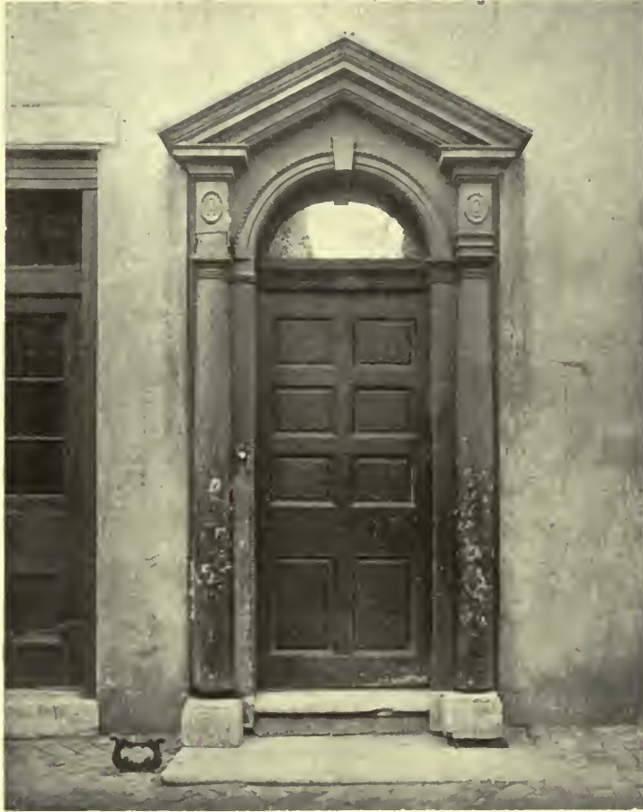
DOORWAY AT 402 WOOD STREET, PHILADELPHIA.
