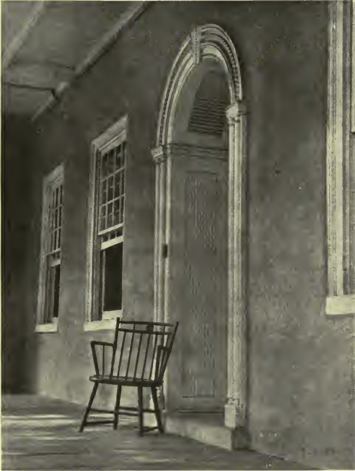
ENTRANCE OF HOUSE AT CHESTER SPRINGS, PA. BUILT BEFORE THE REVOLUTION.
