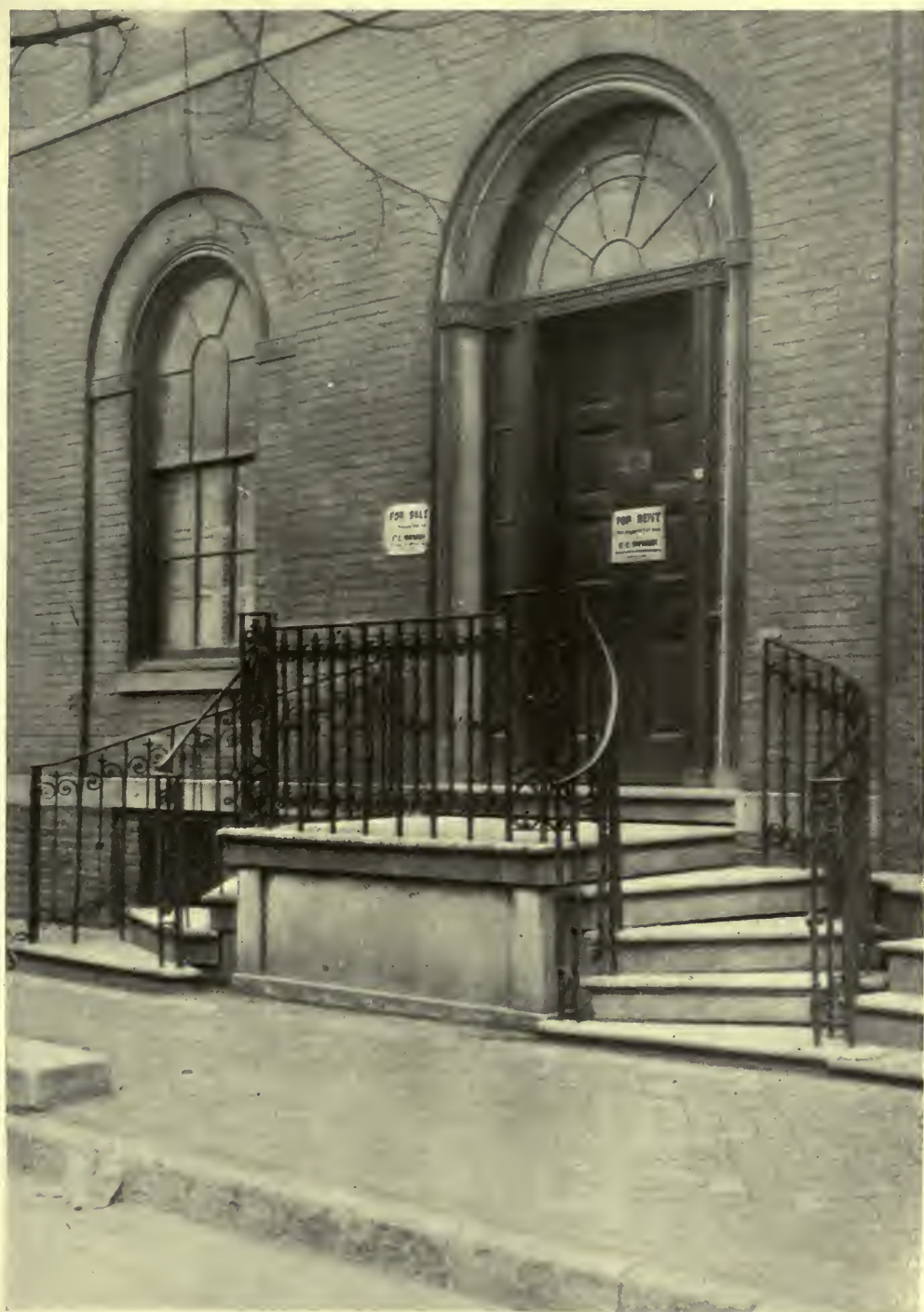
ENTRYWAY OF BELTZHOOVER HOUSE, CARLISLE, PA. EARLY NINETEENTH CENTURY.
