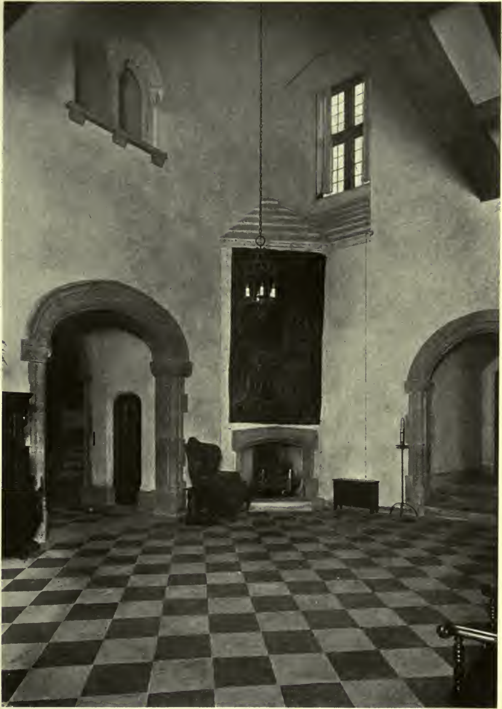
ENTRANCE HALL—RESIDENCE OF WILLIAM R. COE, ESQ., OYSTER BAY, L. I. WALKER & GILLETTE, ARCHITECTS,
