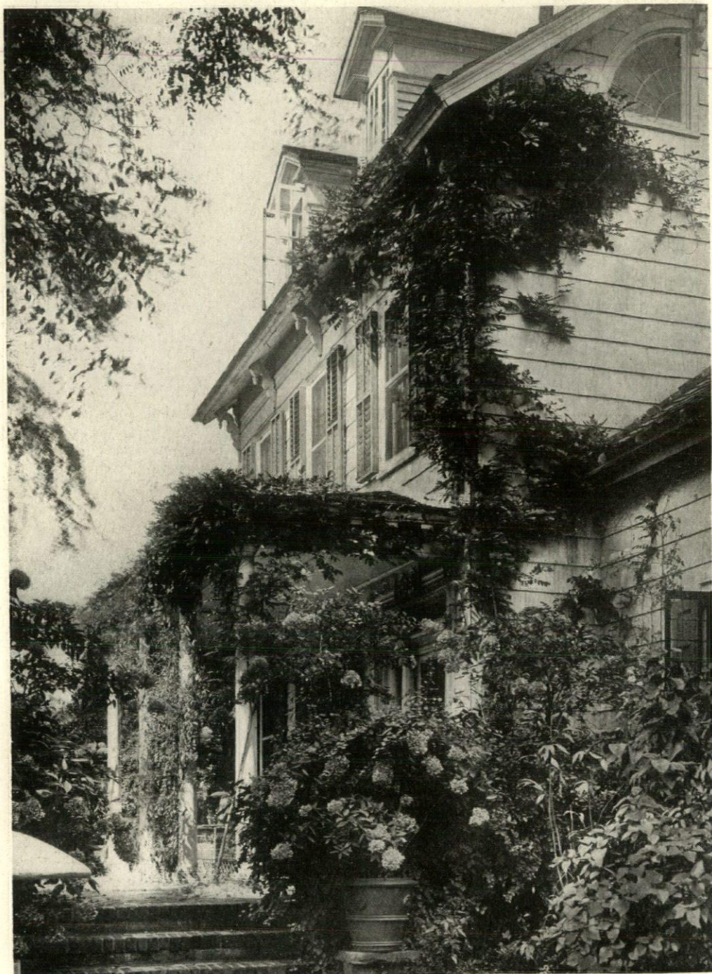
THE LOW PART OF THE HOUSE WAS BUILT IN 1673, AND THE "NEW" PART IN 1795, ALTHOUGH THE DOORWAY WAS NOT PUT IN PLACE UNTIL 1812. ORIGINALLY, THE PORCH HAD A RAILING AND WOODEN FLOOR. THESE WERE REMOVED BY MR. MIZNER, WHO ADDED THE TERRACE, WHICH IS EIGHTEEN FEET WIDE, OR THREE TIMES THE WIDTH OF THE ORIGINAL PORCH.
