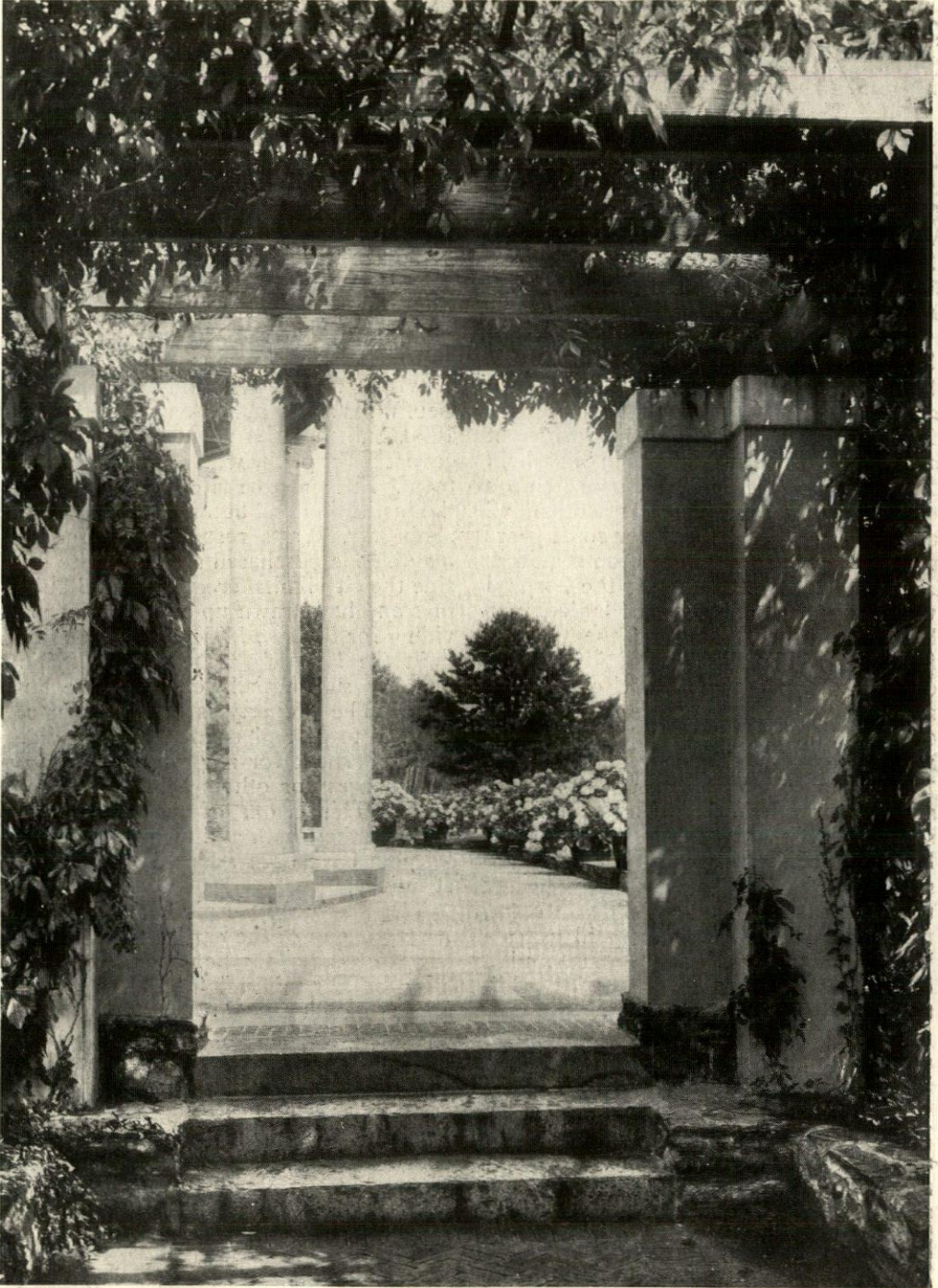
LOOKING THROUGH ROSE ARBOR—RESIDENCE OF GEORGE C. BOWEN, ESQ., PUTNAM COUNTY, N. Y. LA FARGE & MORRIS, ARCHITECTS.
