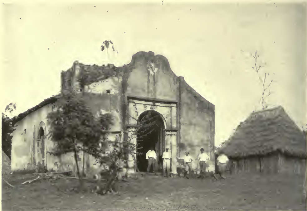
CHURCH AND SCHOOL HOUSE, ARRAJAN, PANAMA.
