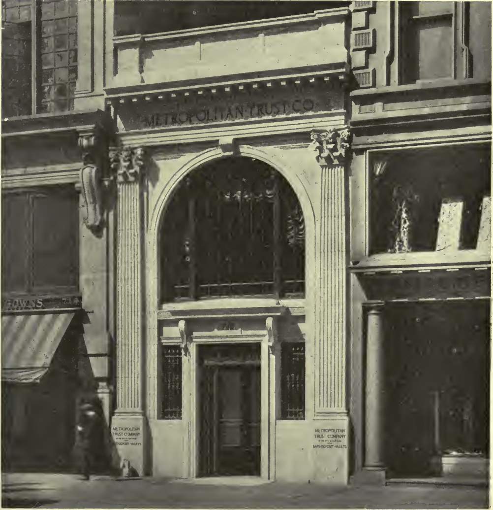
METROPOLITAN TRUST COMPANY'S FIFTH AVENUE BRANCH BUILDING, NEW YORK CITY. HOLMES & WINSLOW, ARCHITECTS.
