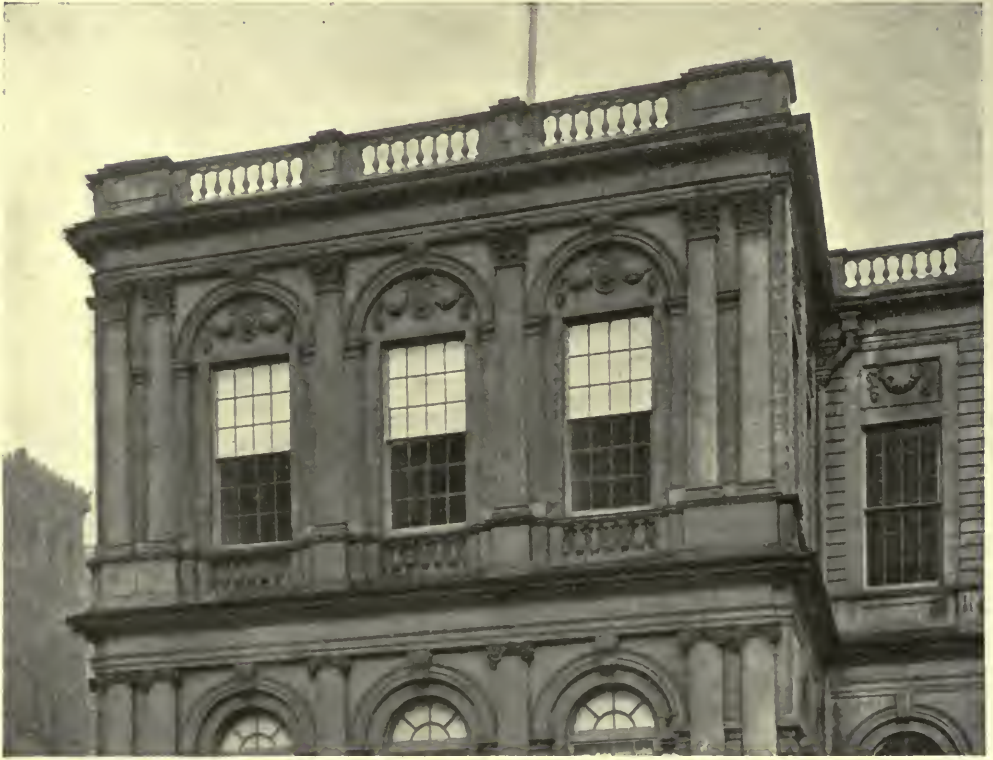
DETAIL AT SECOND FLOOR, SOUTH FRONT.
