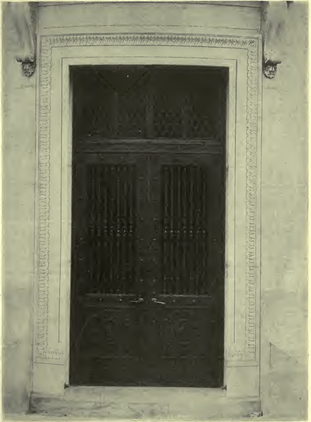
BRONZE DOORS OF CLINIC ENTRANCE—FOR- SYTH DENTAL INFIRMARY FOR CHILDREN, BOSTON. EDWARD T. P. GRAHAM, ARCHITECT.
