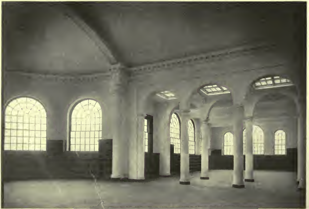
NORTH WING OF MAIN READING ROOM, JOHNS HOPKINS UNIVERSITY, HOMEWOOD, BALTIMORE. Parker, Thomas & Rice, Architects.
