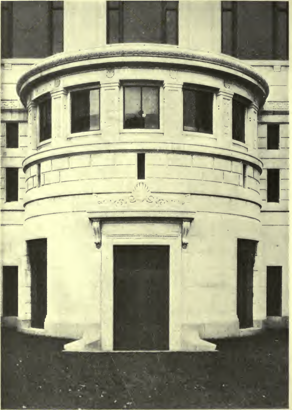
ENTRANCE: TO CLINIC—FORSYTH DENTAL INFIRMARY FOR CHILDREN, BOSTON. EDWARD T. P. GRAHAM, ARCHITECT.
