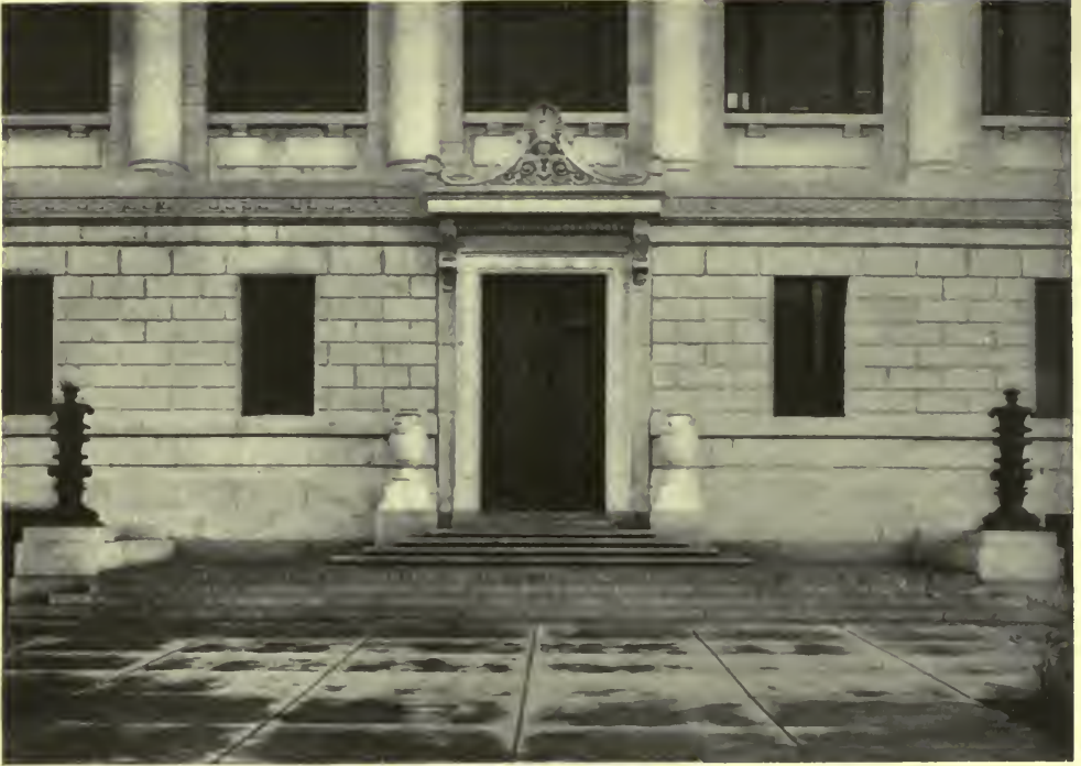
MAIN ENTRANCE—FORSYTH DENTAL INFIRMARY FOR CHILDREN, BOSTON. Edward T. P. Graham, Architect.
