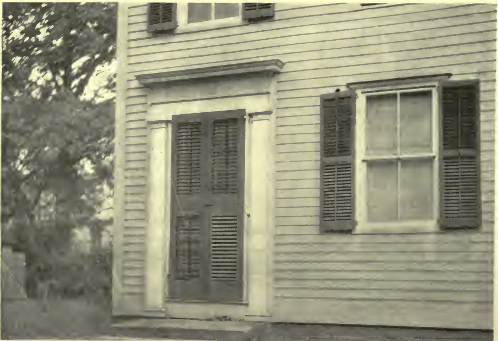
TYPICAL DOORWAY OF SMALL HOUSE OF THE PERIOD OF THE CLASSIC REVIVAL.
