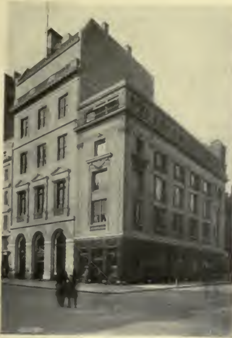
A NEW YORK SHOP, IN AN ADAPTATION OF FRENCH RENAISSANCE ARCHITECTURE.
