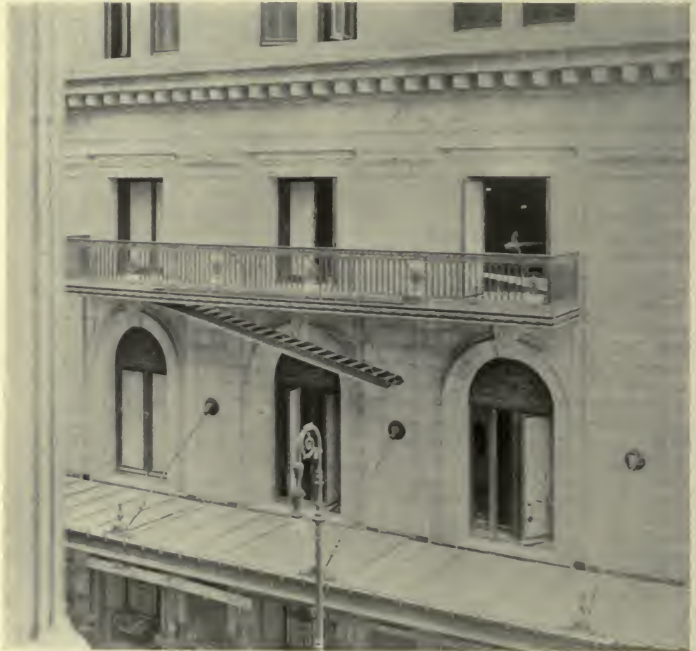
THE BALANCED FIRE-ESCAPE, ÆOLIEN HALL, WARREN AND WETMORE, ARCHITECTS.
