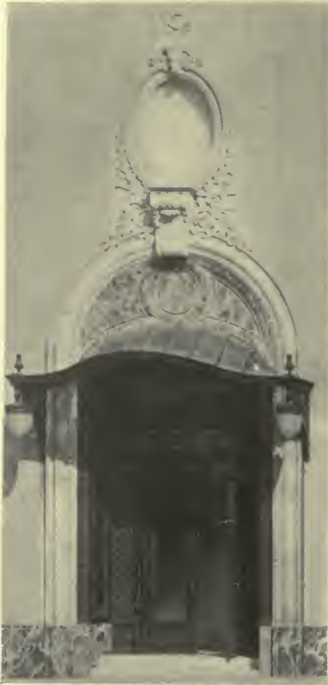
DETAIL OF DOOR (42ND ST. FRONT) ÆOLIAN HALL, NEW YORK CITY. Warren and Wetmore, Architects.
