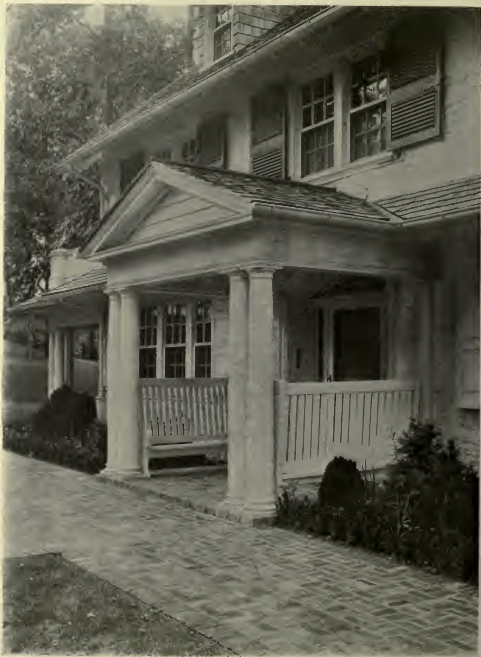
PORCH DETAIL—RESIDENCE OF FRANKLIN BAKER, JR., ESQ., GERMANTOWN, PA. DUHRING, OKIE AND ZIEGLER, ARCHITECTS.
