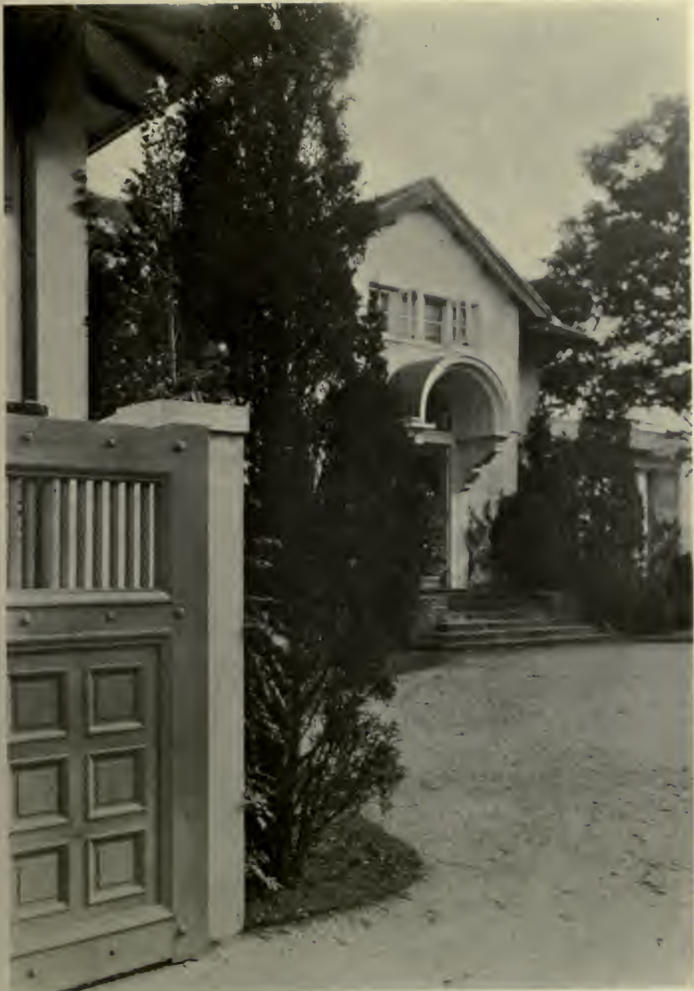
ENTRANCE DETAIL—RESIDENCE OF THOMAS H. KERR ESQ. WHITE PLAINS, N. Y. ALBRO AND LINDBERG, ARCHITECTS.
