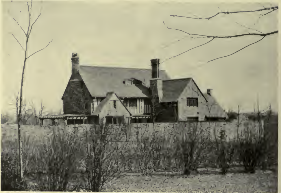
A HOUSE AT CYNWYD, PA. Mellor and Meigs, Architects.
