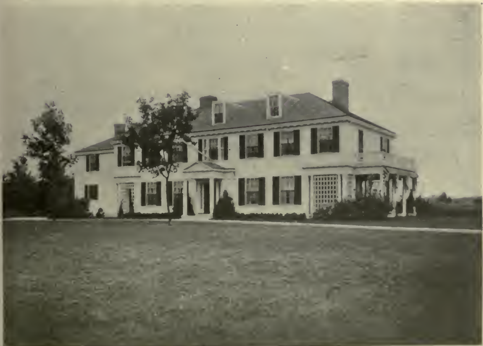
RESIDENCE OF MURRAY BALLOU, ESQ., CONCORD, MASS. Derby, Robinson & Shepard, Architects.
