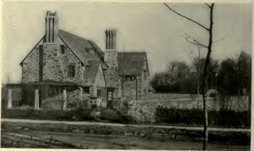
A HOUSE AT CYNWYD, PA. Mellor and Meigs, Architects.
