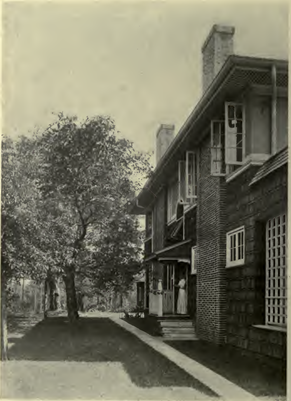
DETAIL, RESIDENCE OF A. H. von BAYER, ESQ., TUSCALOOSA, ALA. W. LESLIE WELTON, ARCH.
