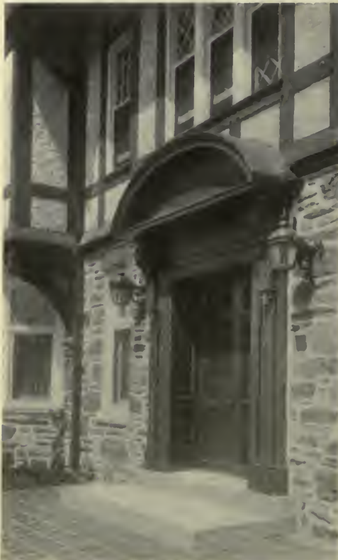
FRONT DOOR DETAIL. RESIDENCE OF GRANVILLE H. LE MAISTRE, ESQ., MERION, PA. D. Knickerbacker Boyd, Architect.
