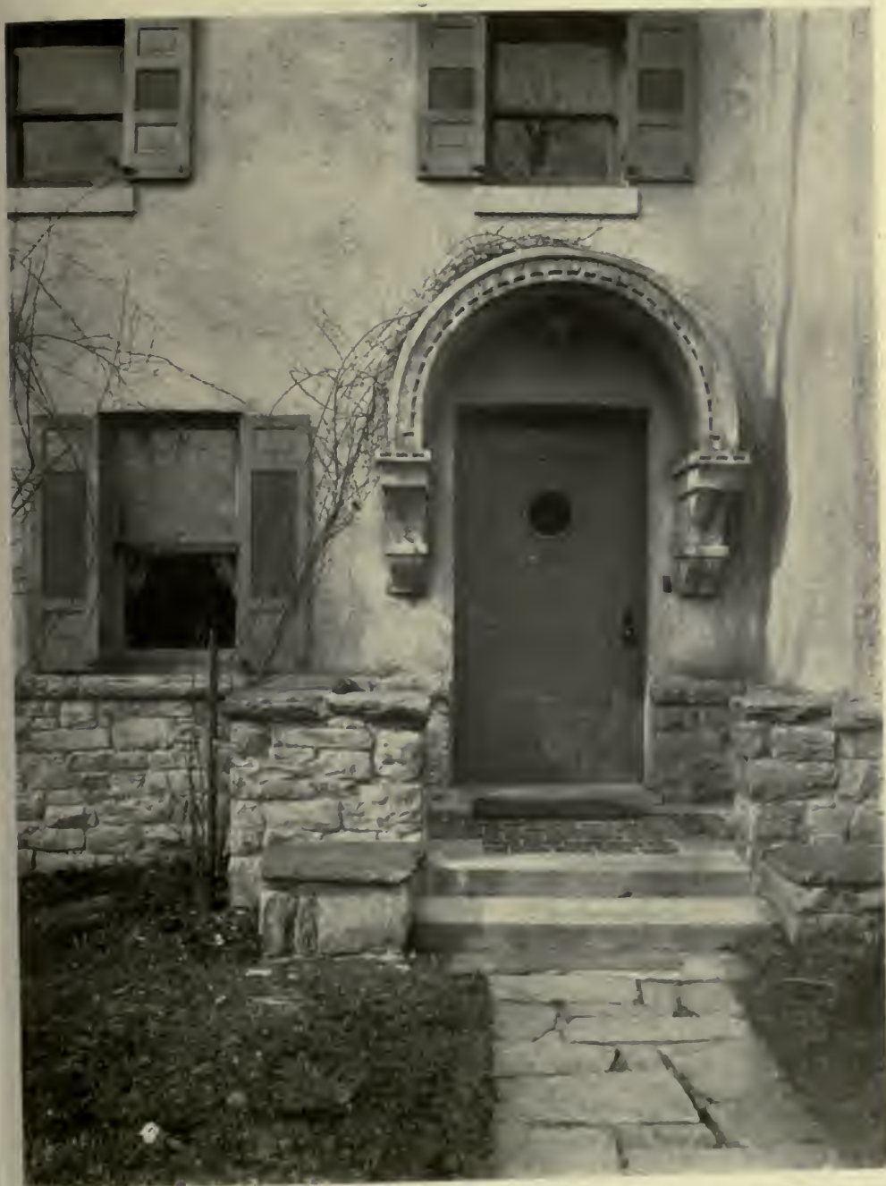
AN ENTRANCE DETAIL—HOUSE AT ROLAND PARK. BALTIMORE, MD. EDWARD L. PALMER, JR., ARCHITECT.
