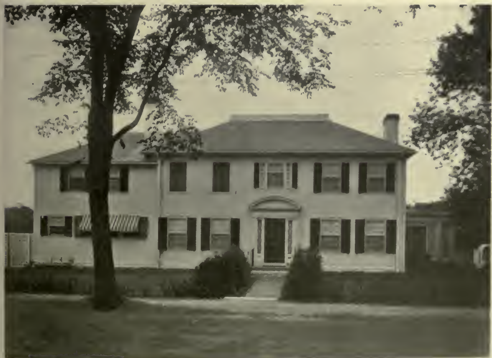
RESIDENCE OF MRS. E. S. BARRETT, CONCORD, MASS. Derby, Robinson & Shepard, Architects.
