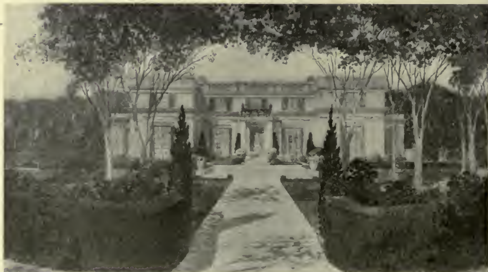
A DRAWING FOR THE RESIDENCE OF J. L. KENDALL, ESQ., PITTSBURGH, PA. Janssen and Abbott, Architects.
