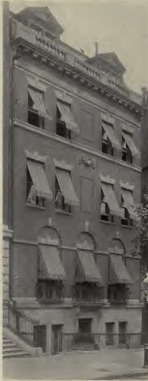
FIG. 9.—754 PARK AVENUE. Geo. H. De Gersdorff, Architect.
