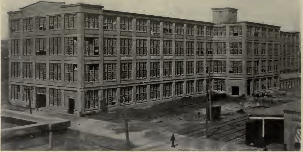
FIG. 4. A REINFORCED CONCRETE FACTORY BUILDING.
