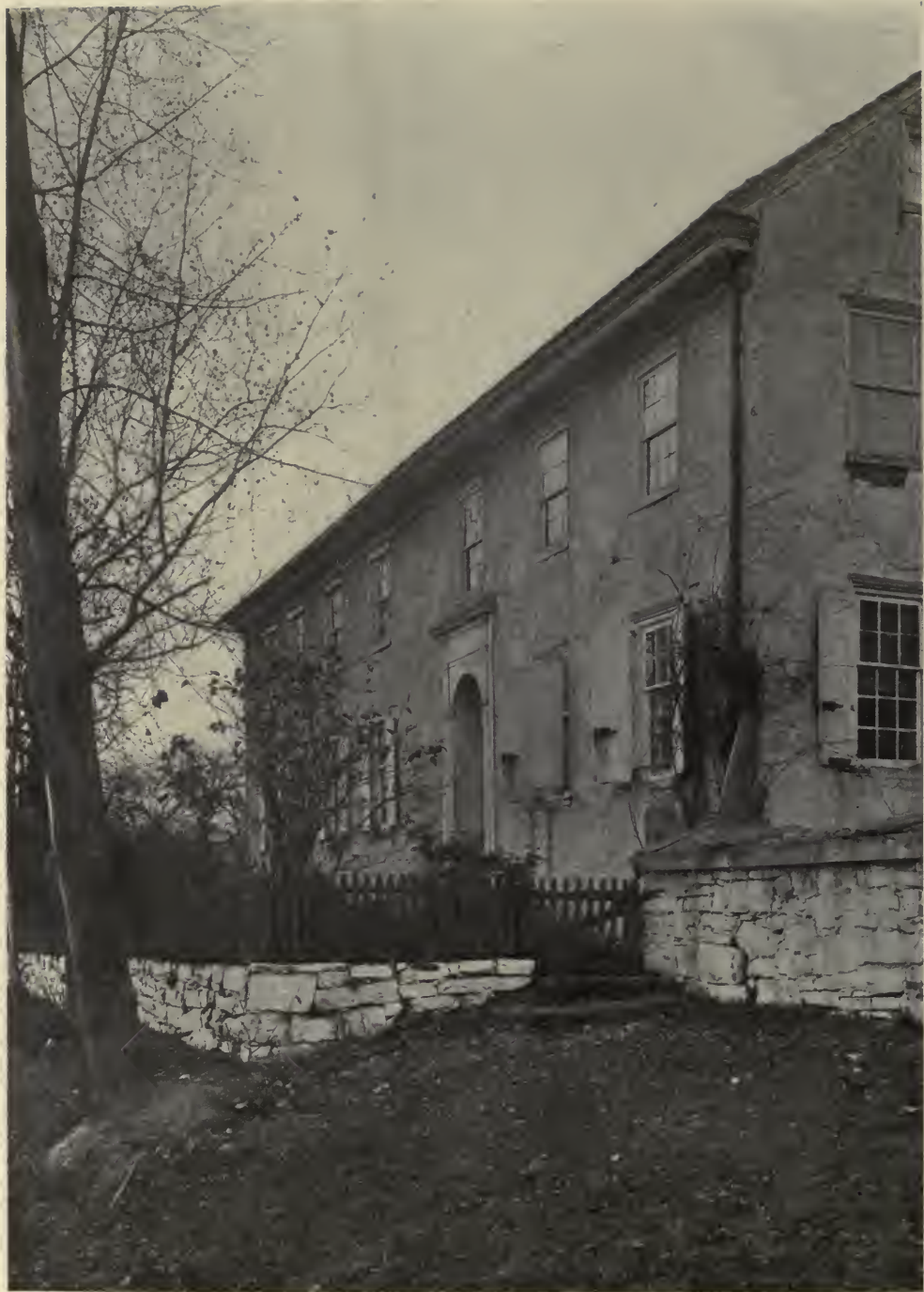
DETAIL OF MAIN DOORWAY AND FRONT OF STUCCO-COVERED STONE HOUSE BEYOND GLASGOW—MOST OF THESE HOUSES, EACH ABOUT 100 YEARS OLD HAS A DELICATELY COVERED WOOD CORNICE IN GOOD CONDITION.
