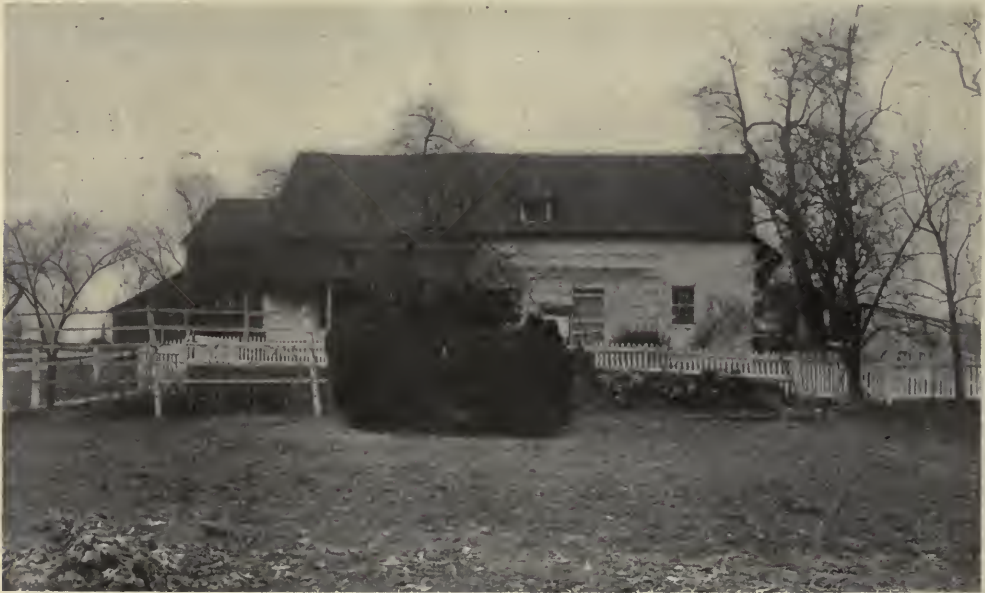
AN 18TH CENTURY HOUSE—THE WALLS ARE OF LOGS WITH A COURSE OF STONE LAID OVER THE TOPS OF THE WINDOWS AND THE WHOLE WHITEWASHED.
