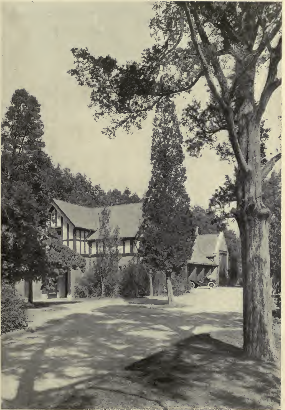
GARAGE—W. J. MATHESON, ESQ. Fort Hill, L. L. Clinton Mackenzie, Arch't.
