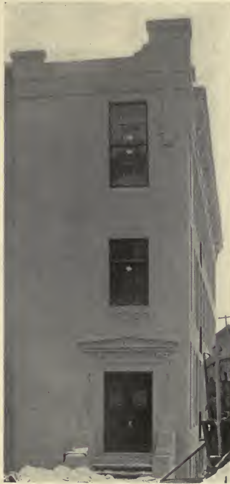
FIG. 6. SKILFUL TREATMENT OF A CONCRETE CORNICE.
