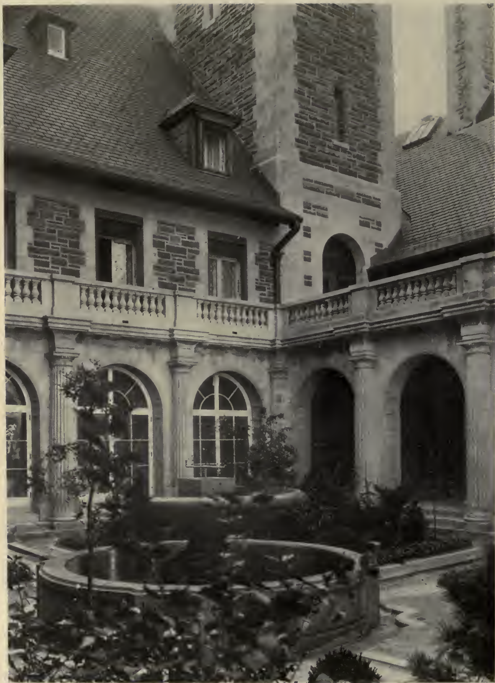
PATIO—RESIDENCE OF MRS. E. H. HARRIMAN, ARDEN, N. Y. CARRERE & HASTINGS, ARCHITECTS.
