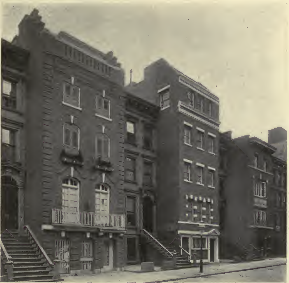
FIG. 13.—NOS. 122-126-130 EAST 80TH STREET. Schwartz & Gross, Architect.
