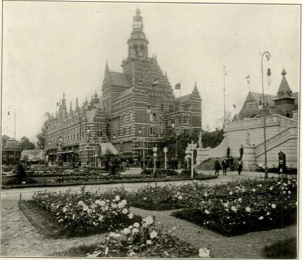
FIG. 11. THE BRUSSELS EXPOSITION, 1910—THE DUTCH BUILDING AND DUTCH GARDEN. W. Kromhout, Architect.
