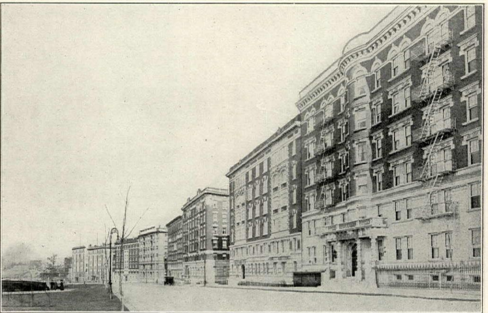
137TH STREET-RIVERSIDE DRIVE, LOOKING NORTH. New York City.
