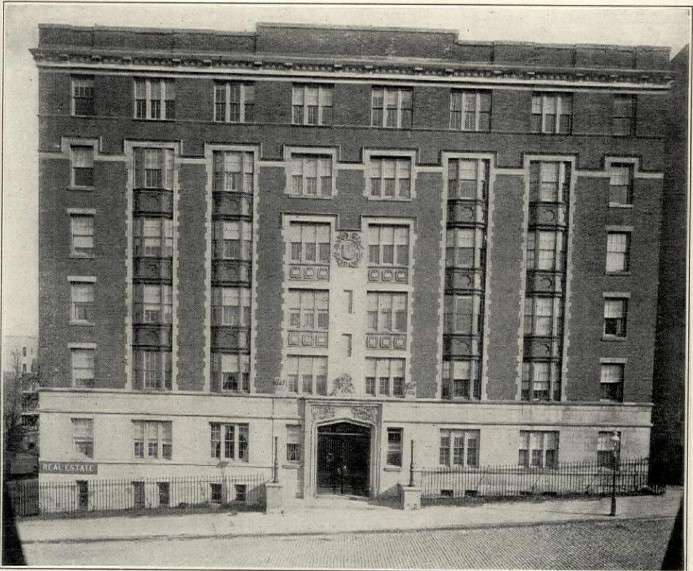
SOUTHEAST CORNER OF 127TH STREET AND RIVERSIDE DRIVE.
