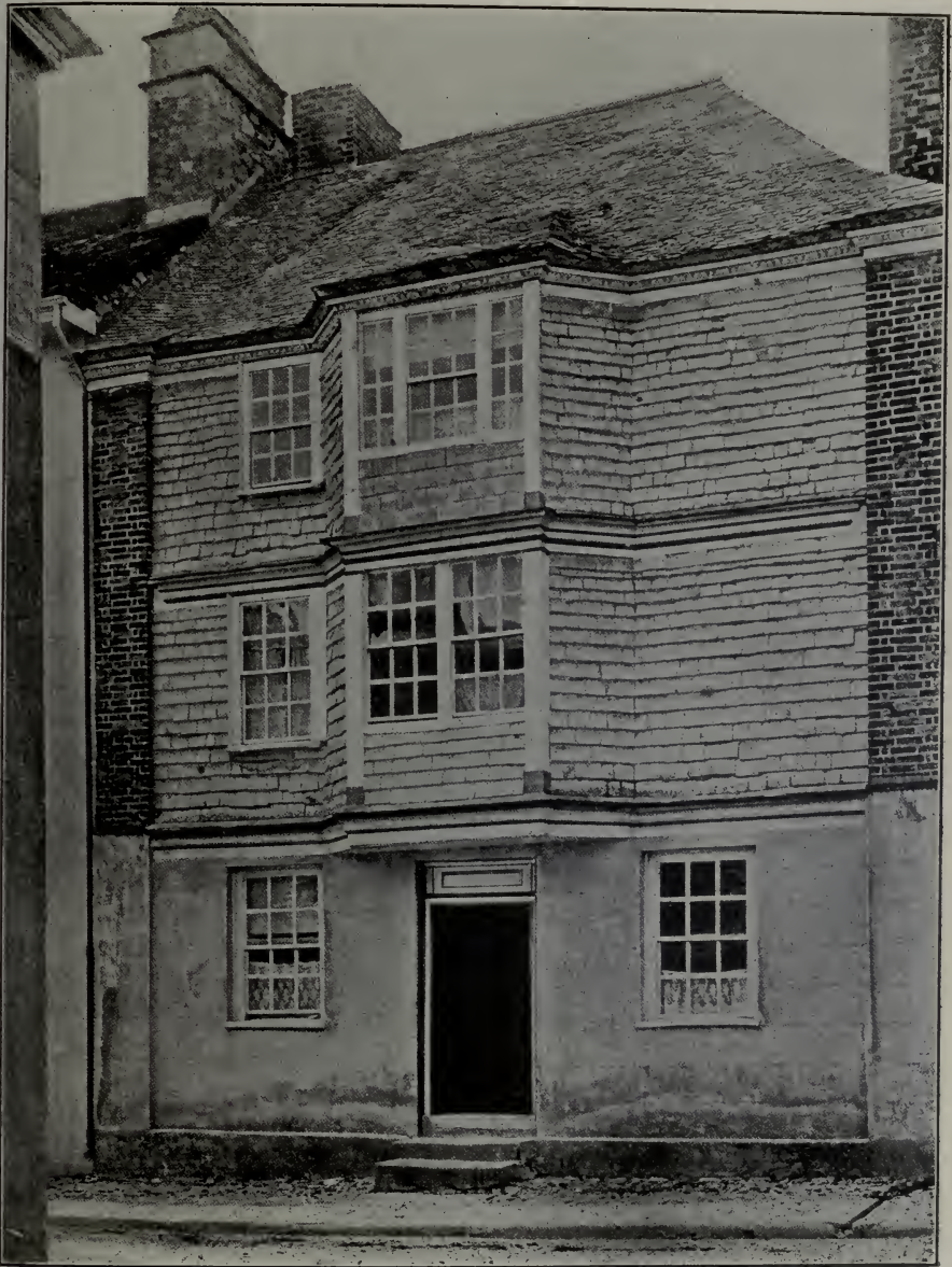
FIG. 10. HOUSE AT ASHBURTON. Slating replaces weather-boarding.
