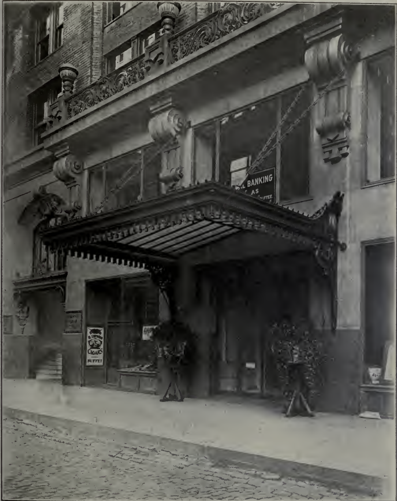
FIG. 7. A WELL-HUNG MARQUISE OF IRON AND WIRE GLASS. THE RECTOR BUILDING. Chicago, Ill.
