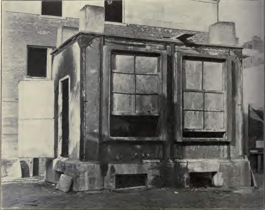
FIG. 1. THE FIRE TEST HOUSE AT COLUMBIA UNIVERSITY, SHOWING THE RESULT OF A FIRE TEST ON WIRE GLASS.
