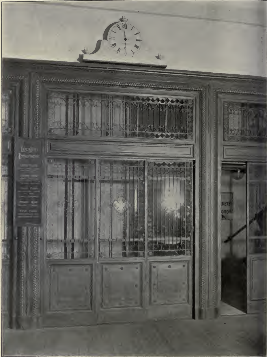
FIG. 6. A MORE ELABORATE METAL DECORATION WITH LESS GLASS SURFACE THAN FIG. CHANDLER STORE BUILDING. Boston, Mass. Peabody & Stearns, Architects
