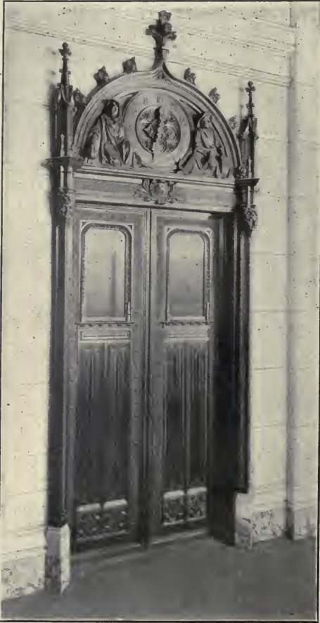
Fig. 3. Bronze and Wire Glass Elevator Doors on the First Story of the Trinity Building, 111 Broadway, New York. Francis H. Kimball, Architect.
