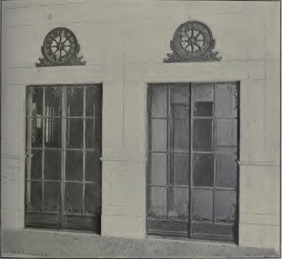
FIG. 5. A FRANK BUT DECORATIVE TREATMENT OF AN IRON AND WIRE GLASS ELEVATOR ENCLOSURE. THE RECTOR BUILDING.
