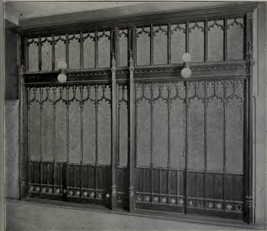
FIG. 4. TYPICAL ELEVATOR ENCLOSURE, 2D TO 23D STORIES, TRINITY BUILDING, 11 Broadway, New York.
