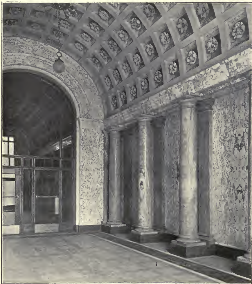
A VERY EFFECTIVE COFFERED VAULT, SHOWING ALSO THE EXTENSIVE USE OF MARBLE FOR STRUCTURAL AS WELL AS FOR DECORATIVE PURPOSES. INDIANAPOLIS COURT HOUSE AND POST OFFICE.
