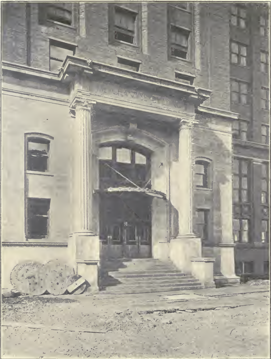
THE MAIN ENTRANCE TO THE MERCHANDISE BUILDING.
