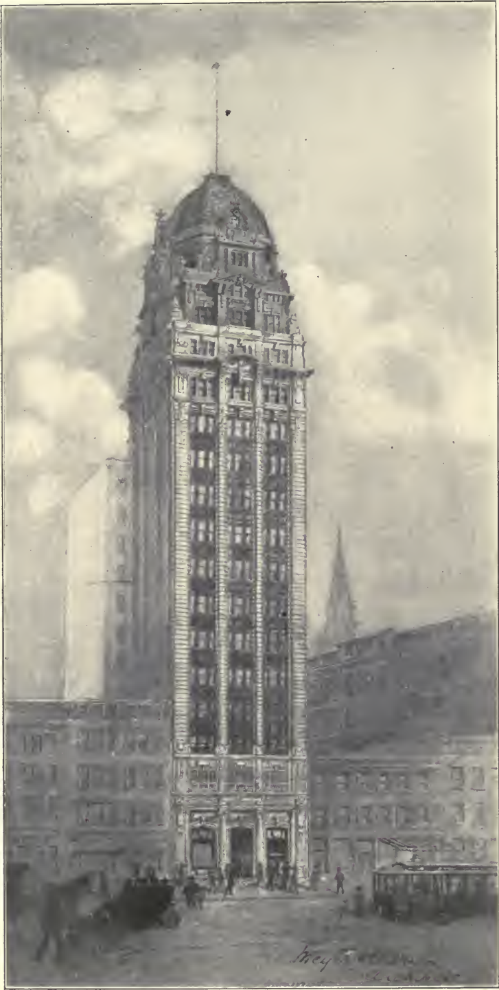
HUMBOLDT SAVINGS BANK BUILDING. San Francisco, Cal. Meyer & O'Brien, Architects. Now in course of construction.
