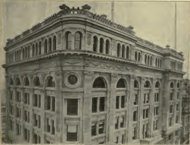
UPPER STORIES OF MUTUAL LIFE INSURANCE COMPANY'S BUILDING. Nassau Street, New York City. Clinton & Russell, Architects.
