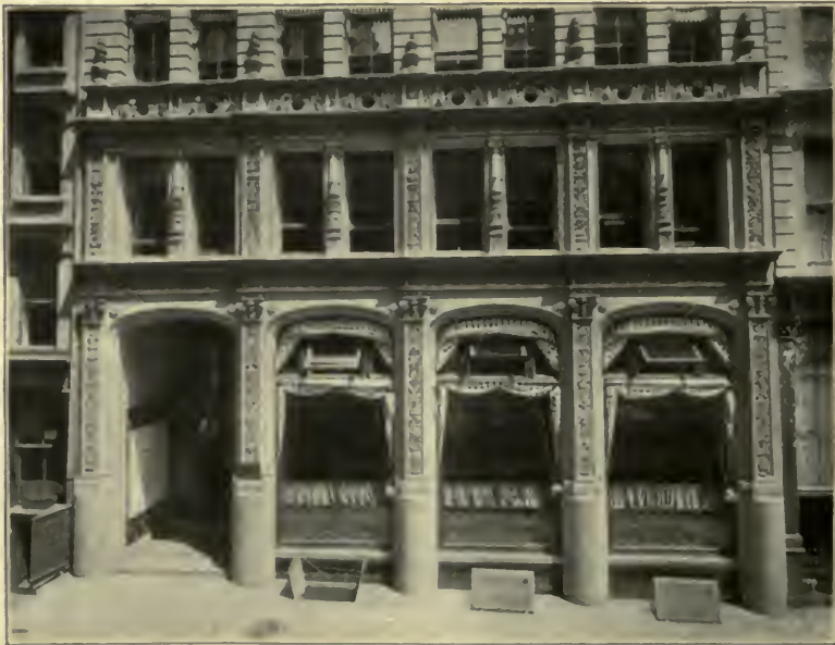
ENTRANCE OF FAHYS BUILDING.
